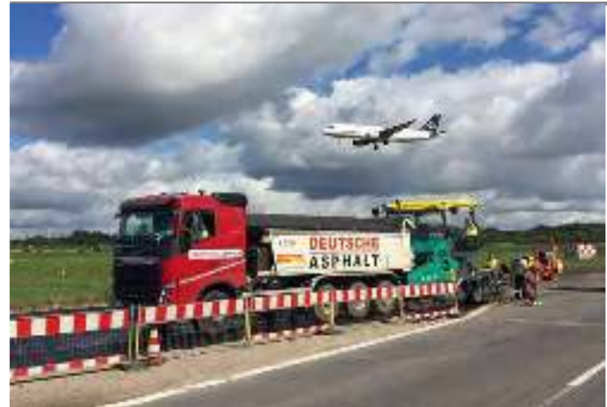
Asphalt installation while airport operations continue without restrictions from air-traffic control's radar
