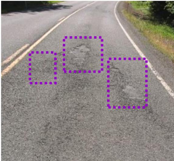
Fig. 2. Consequences of temperature segregation can be road damages such as crumbling, cracks, ruts and potholes (Photo: Sebesta et al., 2013).
